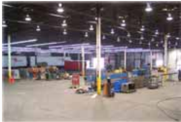
CDS's 30,000 square-foot wing is expected to be completed by the early summer of 2007.
